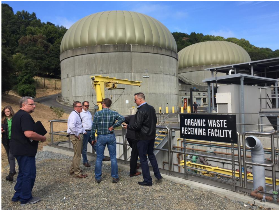
CMSA Treatment Plant Manager Chris Finton explains codigestion process
