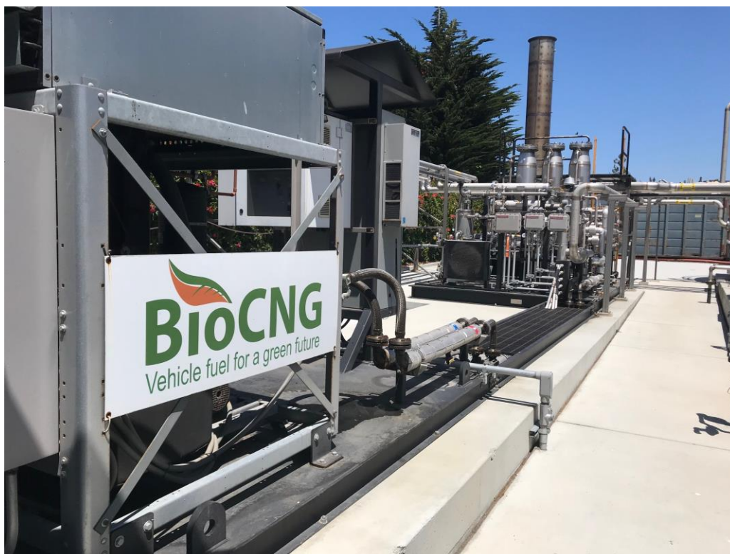
Clean biogas from dry AD process provides CNG for South San Francisco Scavenger fleet
