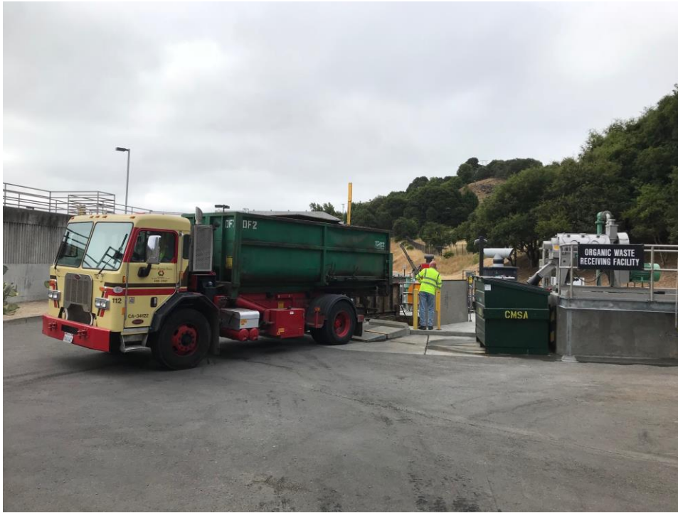
Seven tons of slurried food waste is delivered from MSS to CMSA and blended with 10,000 gallons of FOG daily
