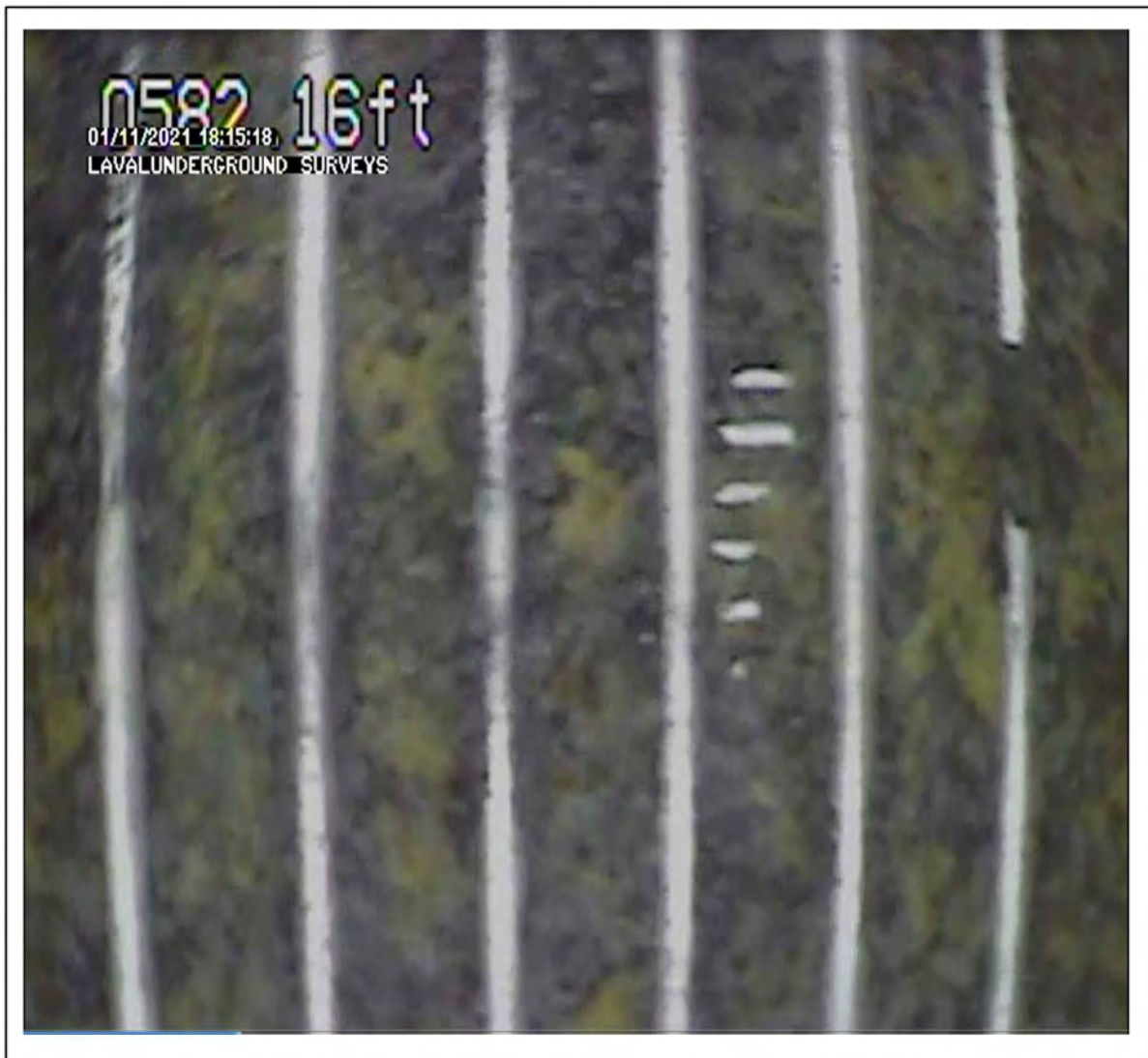
Figure C-2. Examples of Biofouling in Screened MAR Wells.
