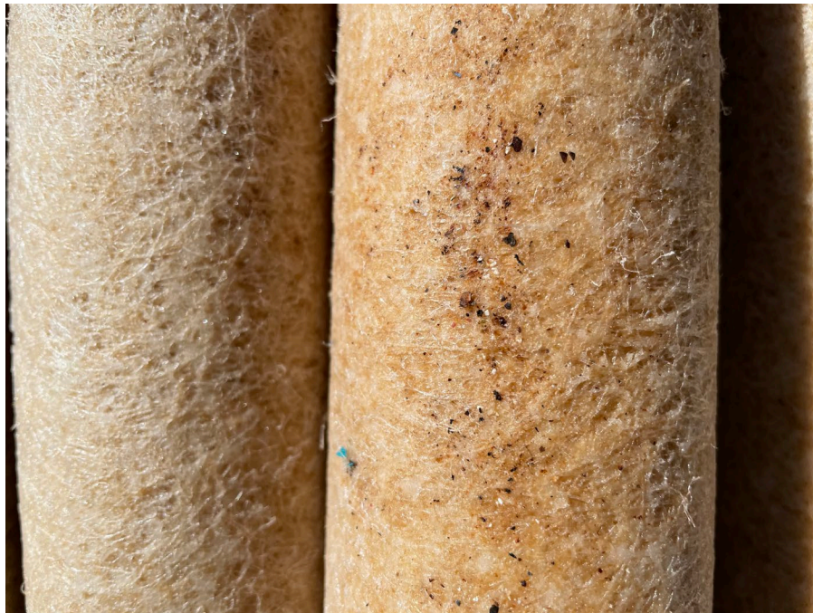
Figure 5-5. Cartridge Filters After Changeout on October 29, 2020.
