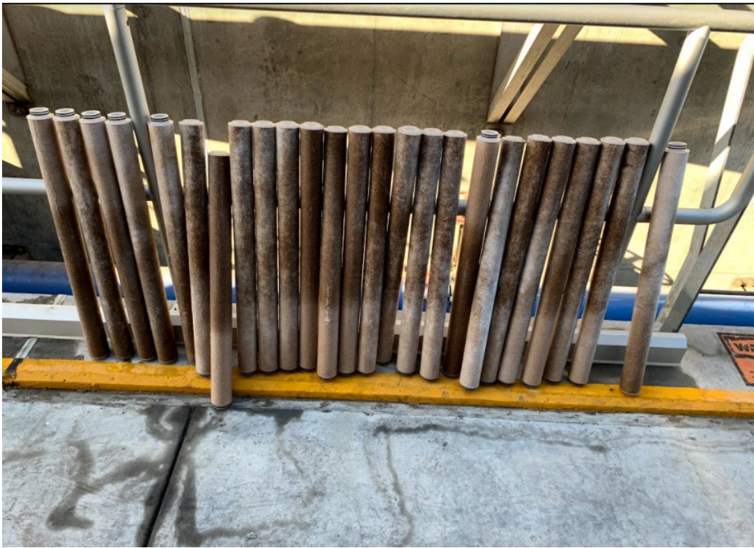
Figure 5-4. Cartridge Filters After Changeout on December 18, 2020.
