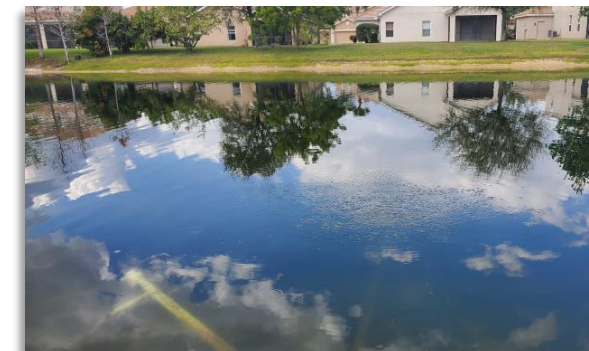
1-Month After Install
