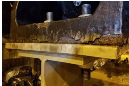
Carbon steel cradle on top of stainless steel base
