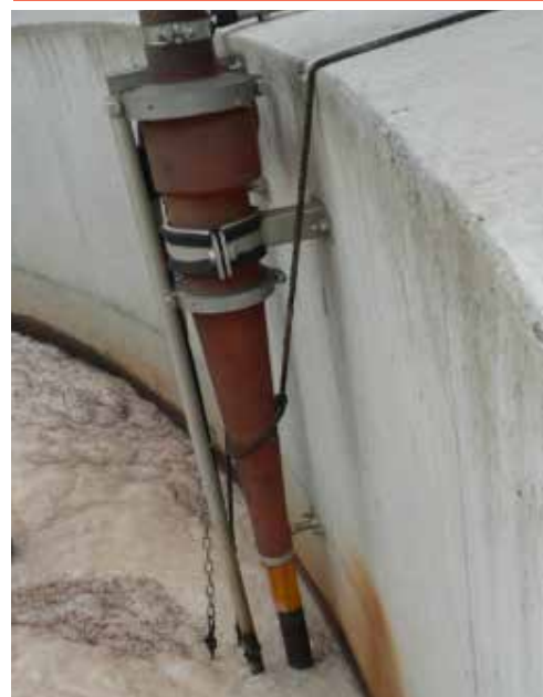
Hydrocyclone retains anammox and washes out competing bacteria.
