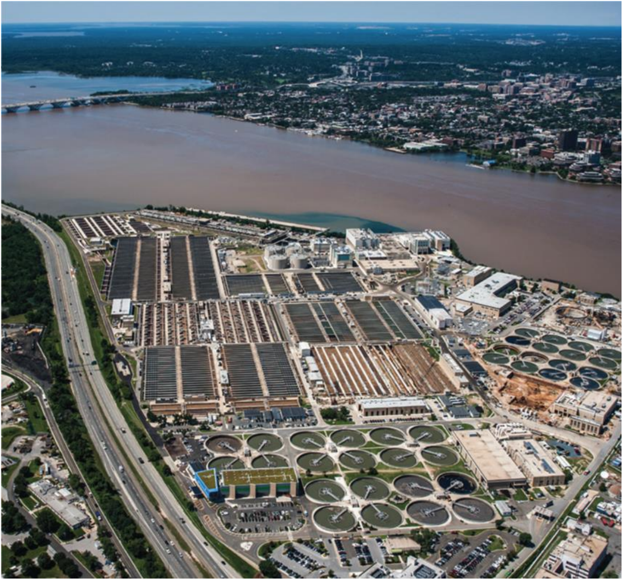
Figure 1 Blue Plains Advanced WWTP (BPAWWTP).
