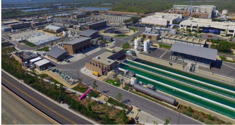
Michelson Water Recycling Plant
